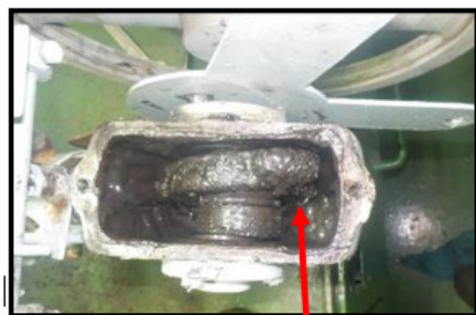
Deteriorated Oil Condition & Damaged Connecting Rod Bearing
