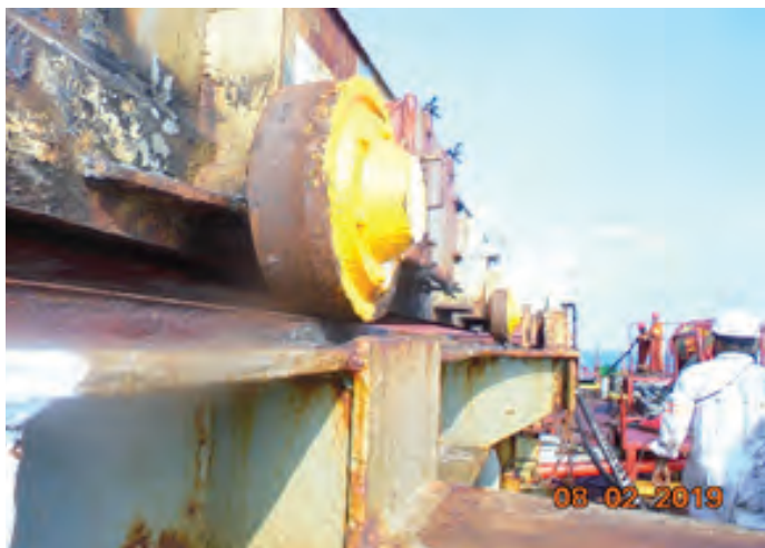
Hatch cover rolled out of the trackway
